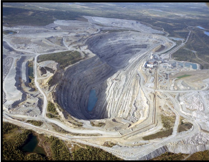
Figure 74: The huge open Pit with a length of 3km and a width of 1km and a depth of about 420m
